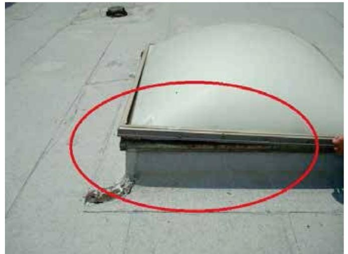
Also, over time the plastic domed panels can become brittle and very susceptible to cracks.
