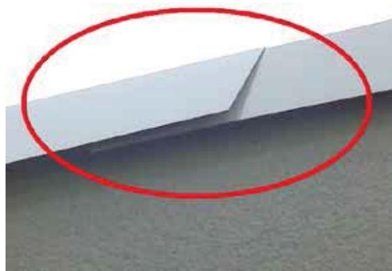
**Tears in the roof cover**, or worn or cracking seams, can allow water to enter below the cover.
